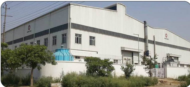
Manufacturing Plant -3 Makino Auto Industries Pvt. Ltd. OEM Business Center and Corporate Office Noida- Uttar Pradesh
